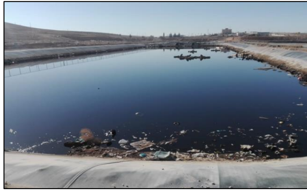
Figure 1: Leachate ponds in Al-Ghabawi landfill (Source: the author).
